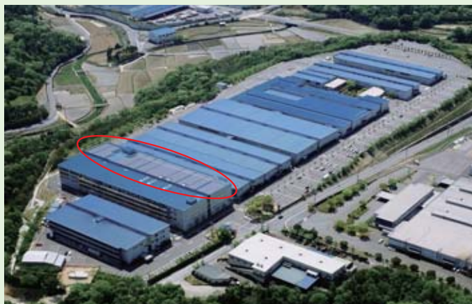
Solar power system
