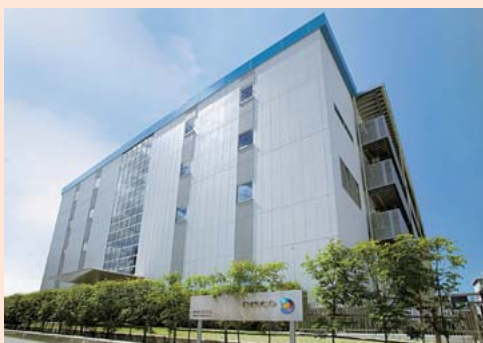
The precision processing tooling building at the Kure Plant
